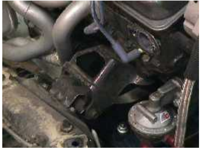
Figure 3: Right Side Motor Mount Installed
